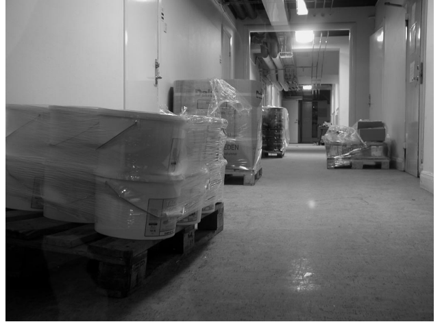
Fig. 6. A cluttered corridor in our institute. These types of obstructions do not pose any problems for navigation and map building.
